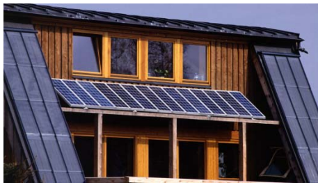
High Performance Buildings
